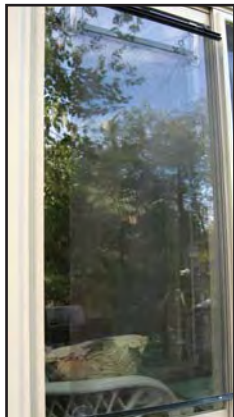
This window is covered with a Bird Screen, which has a cushioning effect if a bird does strike it.
