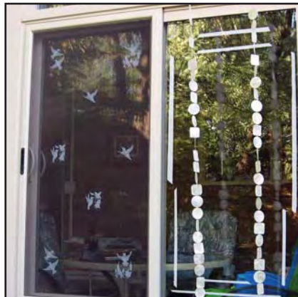
This photo shows two bird collision-prevention treatments. The window at left is covered with decals and also has a screen. The window at right has tape on the outside and strings of shells that move in the wind. Both make this window visible to birds.
